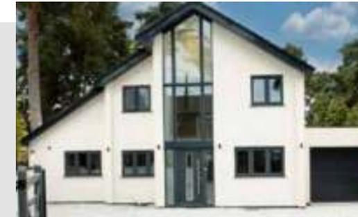
K Mono is a monocouche render, designed for use with render spray machines. It acts as a one coat / one pass finish over most moderate to low strength brick and block work, providing a labour-saving and cost-effective solution due to reduced application times.
